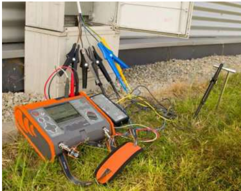
Earth resistance measurement with the AMPI-525 in the field
