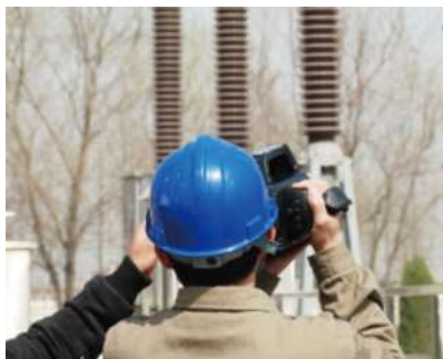
Substation survey with the installation in service
