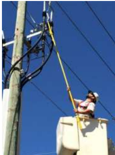
Checking an overhead-line accessory with an insulated hotstick
