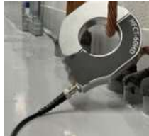
HFCT-HD clamp on the ground return of a cable
