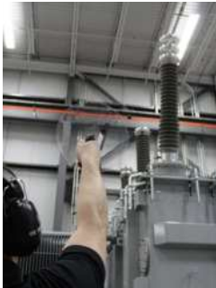
Inspection with the external parabolic sensor at a substation
