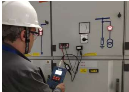
Partial discharge measurement at a transformer substation
