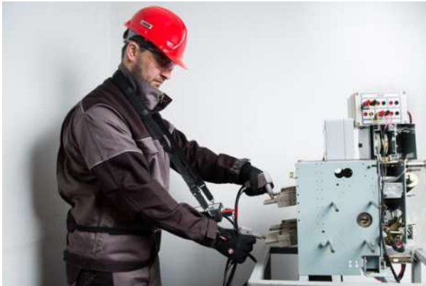
Contact resistance measurement on a breaker at the substation
