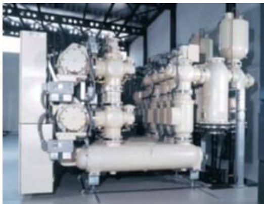
Gas-insulated switchgear, a typical AGRU-8 application
