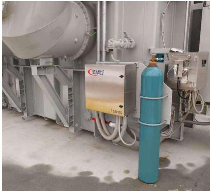
E Series installed on a power transformer
