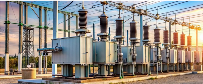
Permanent monitoring of the transformer fleet, with no site visits to draw oil samples.
